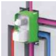
3. Use screws to install plastic boxes.
